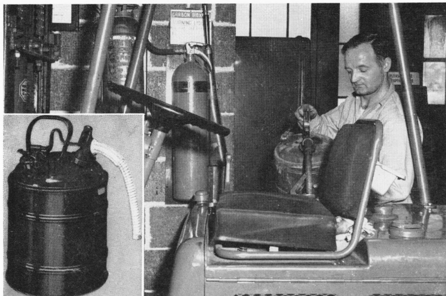
Gus Fabiani, Shell Department, demonstrates the right way to pour gasoline into a lift truck which has "gone dry" away from a pump station. The insert shows the correct safety can provided for this purpose.
